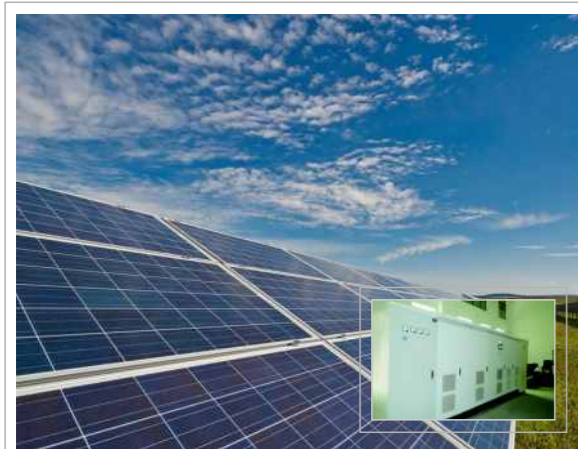
16MW, Shanghai, China
